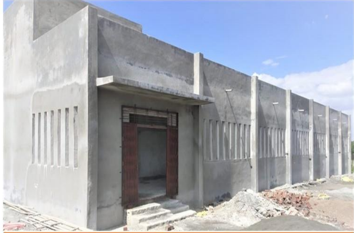
LBI Centre New Building under Construction .
